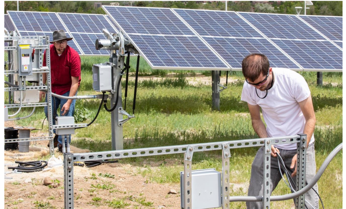
Ongoing maintenance at an agrivoltaics array (Photo credit: Wemer Slocum, NREL)
