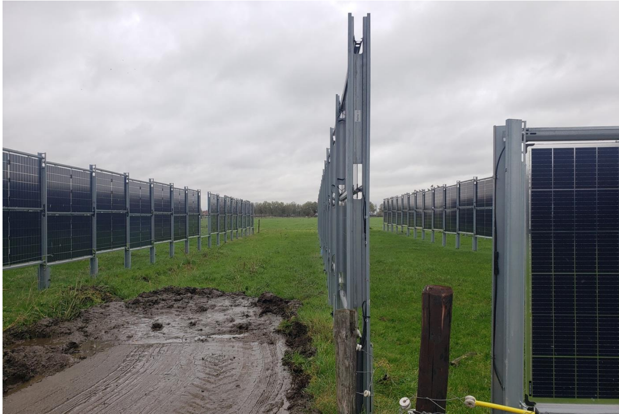
Vertical bifacial agrivoltaic array used for cattle and sheep grazing (Photo credit: Brittany Staie, NREL)
