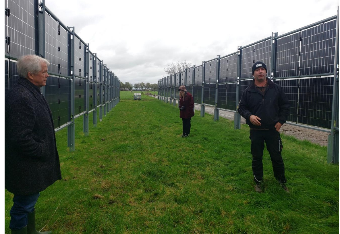
Farmer speaks about integrating cattle into their vertical bifacial array in the Netherlands (Photo credit: Brittany Staie, NREL)
