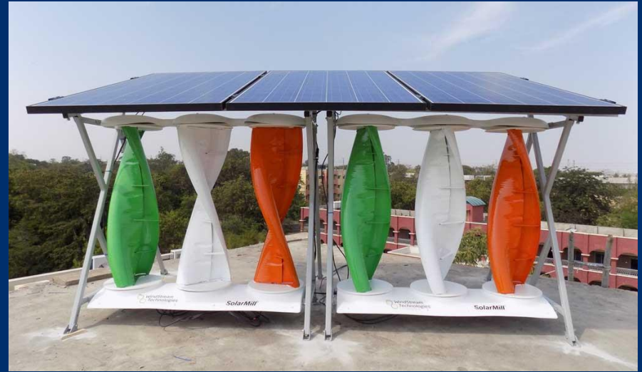
Roof-Top Wind & Solar Hybrid Energy System
