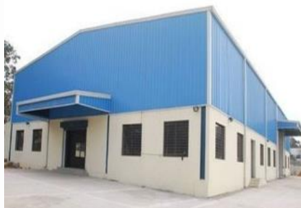
FIGURE 3-44: METAL STRUCTURE TO COVER CHARGING STATION
