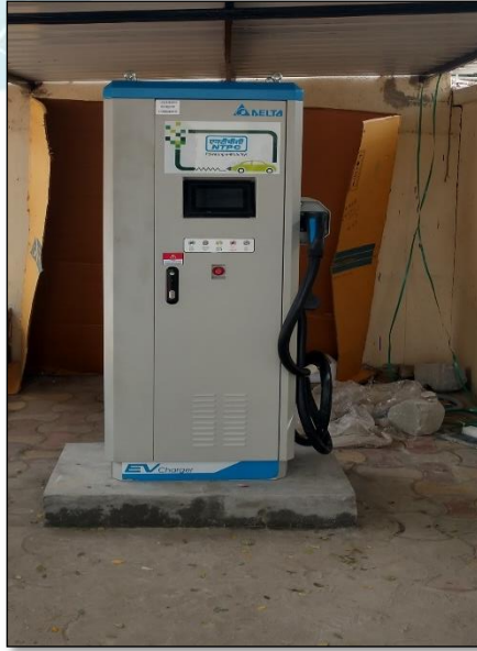
FIGURE 5-1: FLOOR MOUNTED CHARGING STATION
