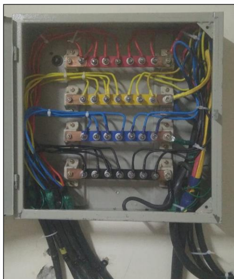
FIGURE 5-3: PROPERLY WIRED BUSBAR
