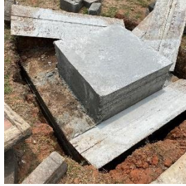
FIGURE 3-45: FOUNDATION TO MOUNT CHARGING STATION
