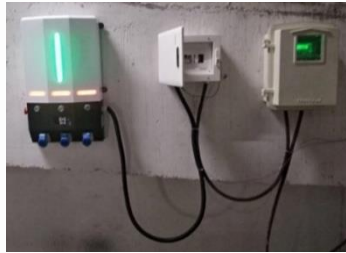
FIGURE 3-46: EXAMPLE PROPER CABLING
