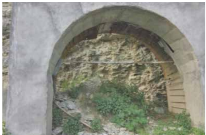
Half-finished construction of a tunnel near Mauwaphant
