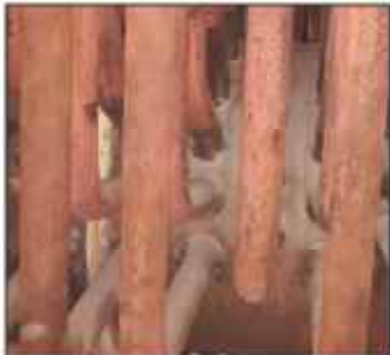
Figure 7 (a)SH Stub (normal)
