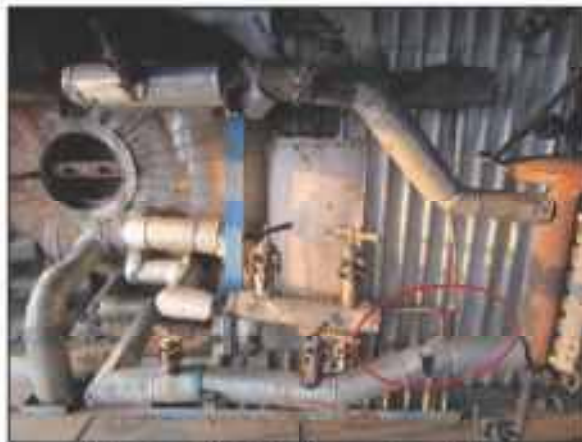
Figure 13: Drain line connections
