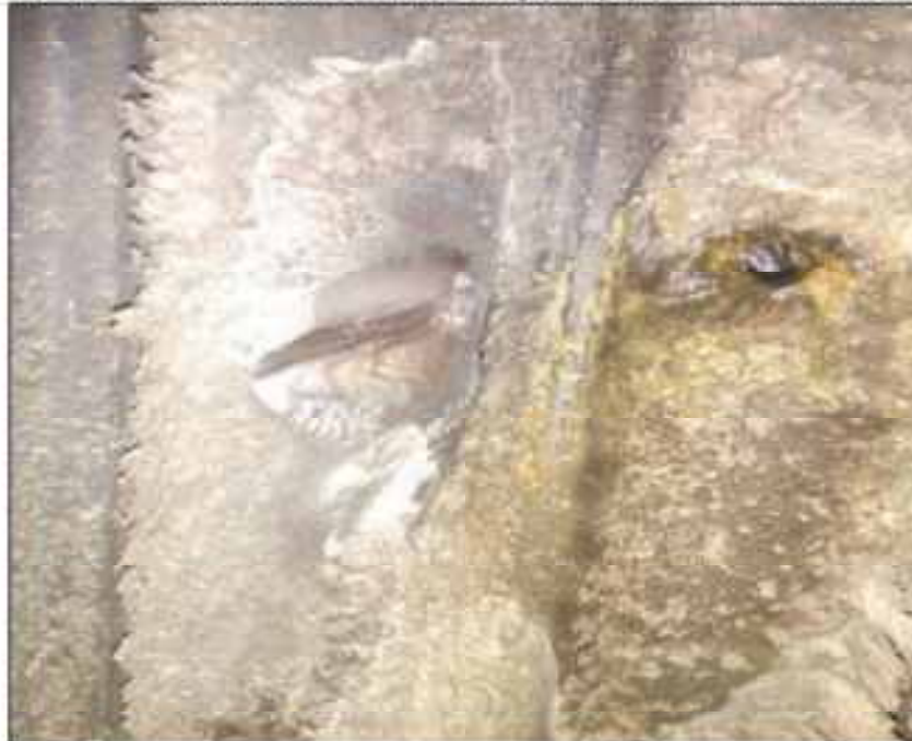
Figure 26: WW hydrogen damage
