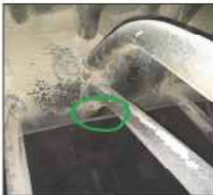
Figure 8: Hanger stub joint
