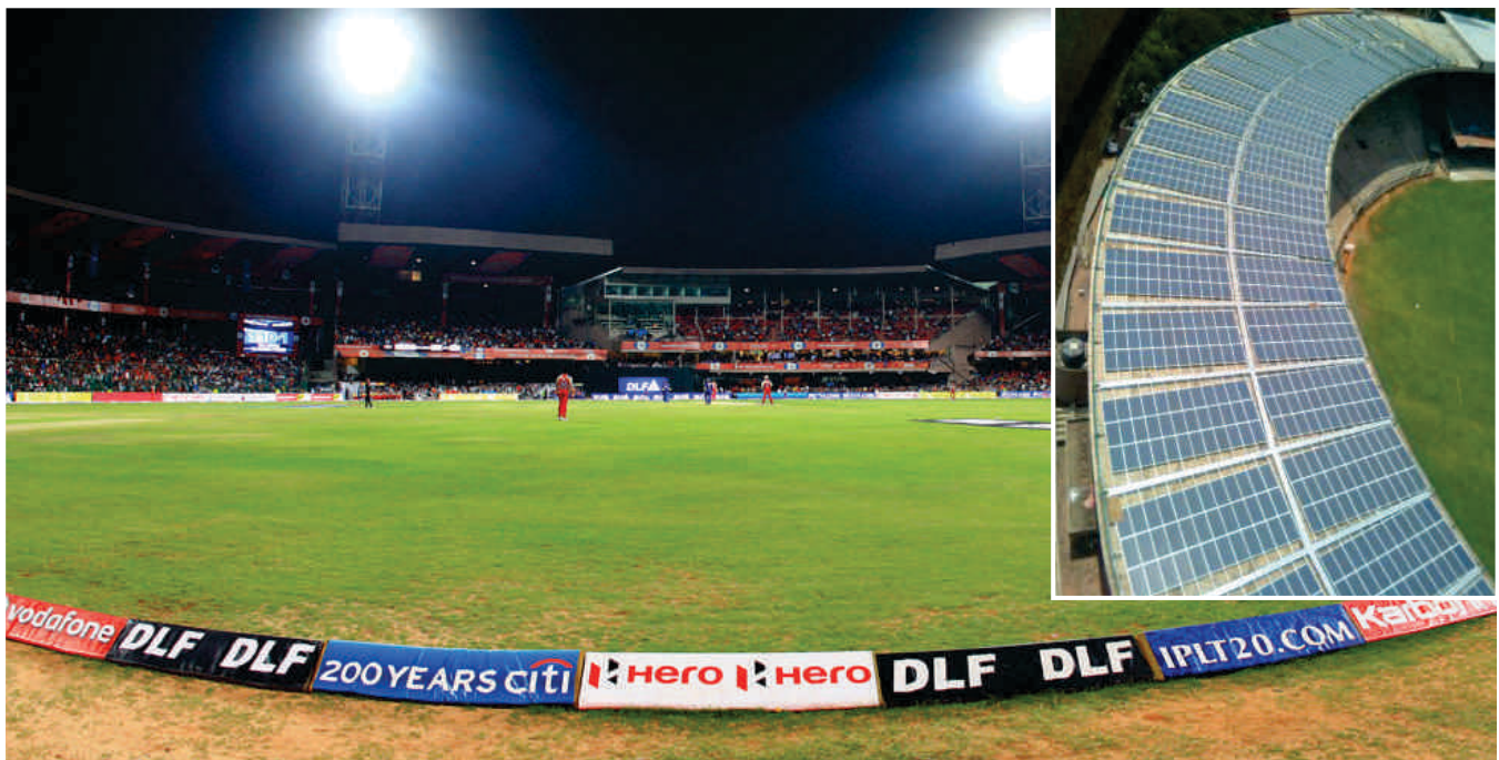
Solar Rooftop Project at Chinnaswamy Cricket Stadium
