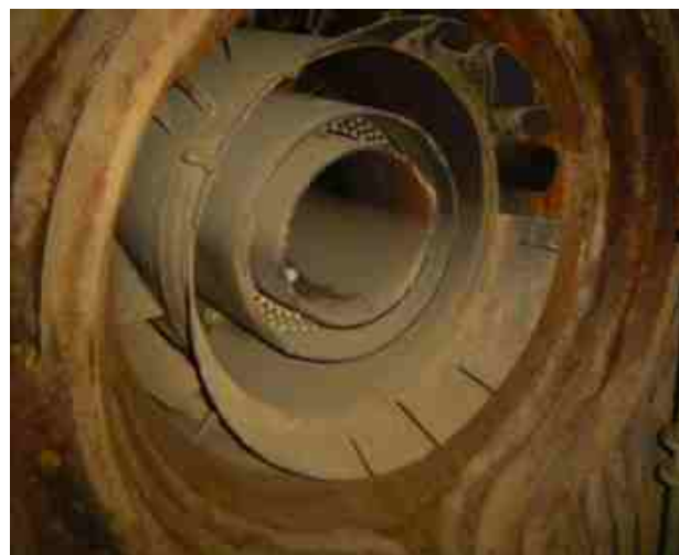
6-71: Ultra Low NO x Burner with Four Air Zones
