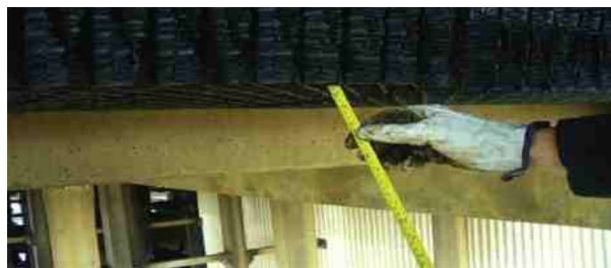
Figure 7-13: Fill Cleanliness Assessment with Tape Measure [6].
