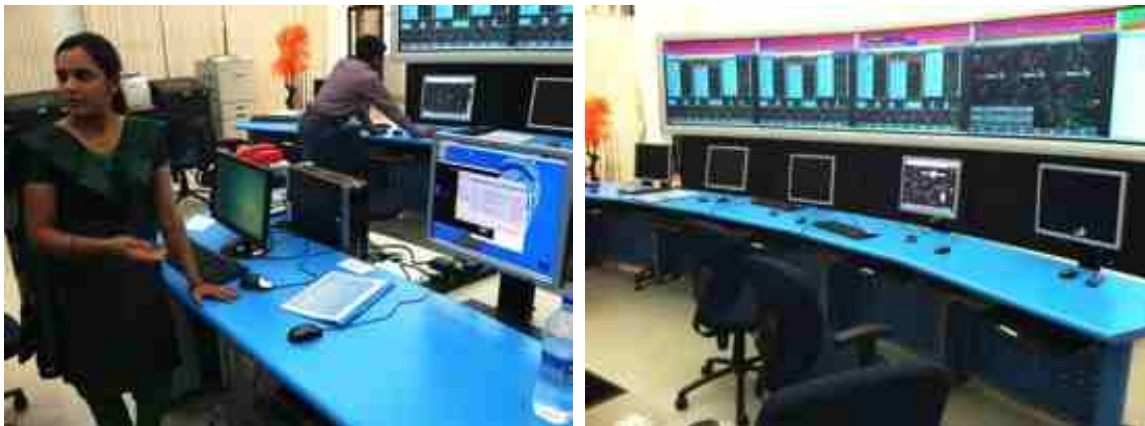
Figure 6-4: World Class Training and Operations Simulation Program at SIPAT Thermal Plant
