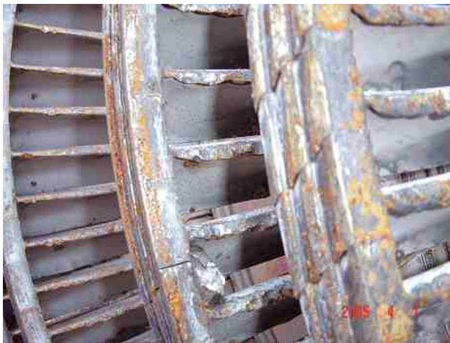
Figure 7-7: Catastrophic SCC Turbine Failure
