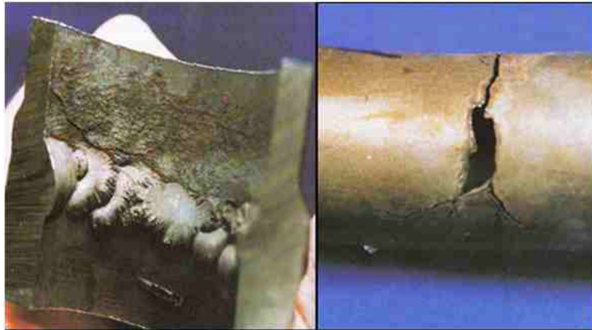
Figure 9-34: Stress Corrosion Cracking
