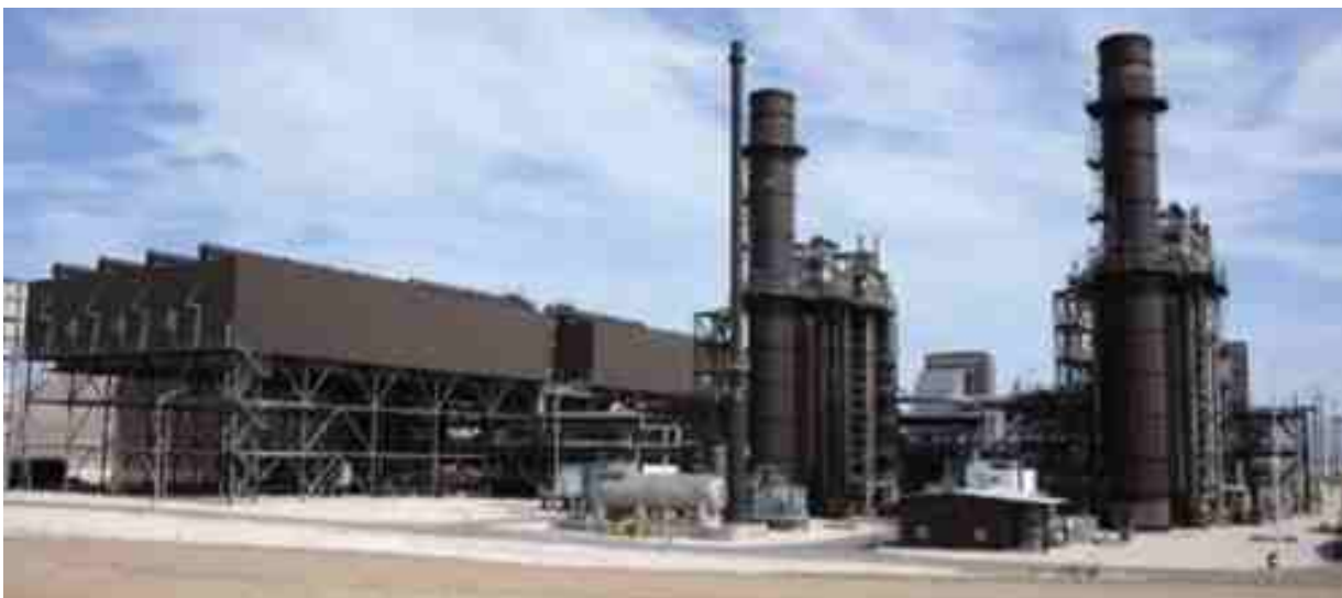
Figure 4-8: Energy's Walter M. Higgins Generating Station in Southern Nevada, USA 530-MW Combined Cycle Power Plant
