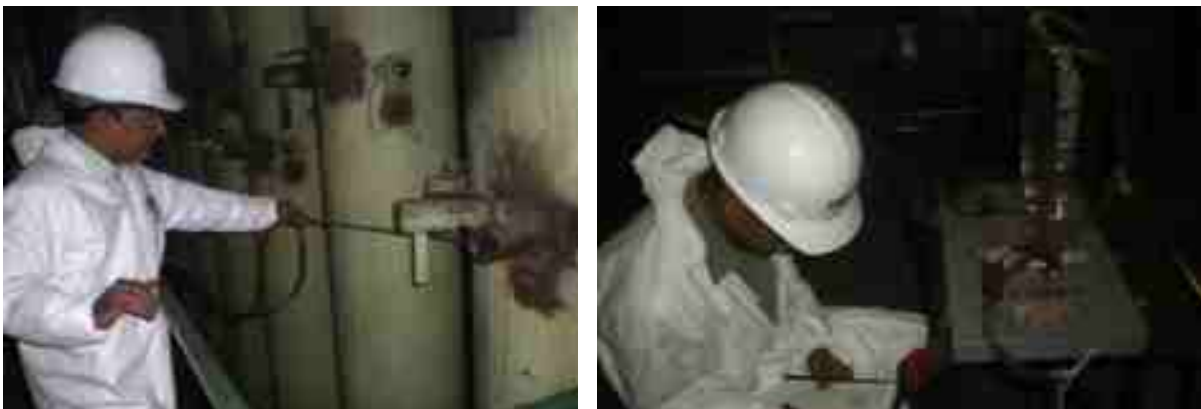
Figure 6-37: Plant Engineers Conducting a Fuel Line Clean Air Test
