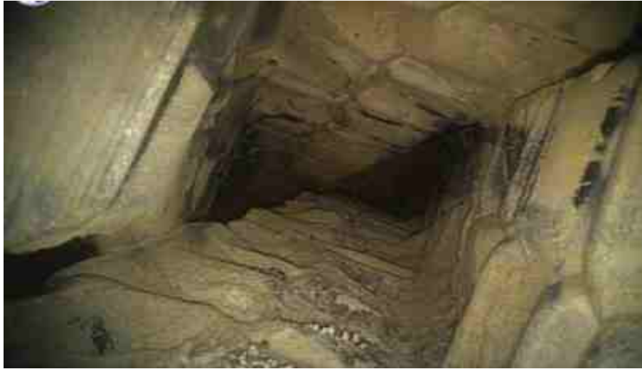
Figure 7-14: Fill Cleanliness Assessment with Boroscope [6]
