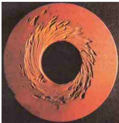
Figure 9-35: Flow Accelerated Corrosion
