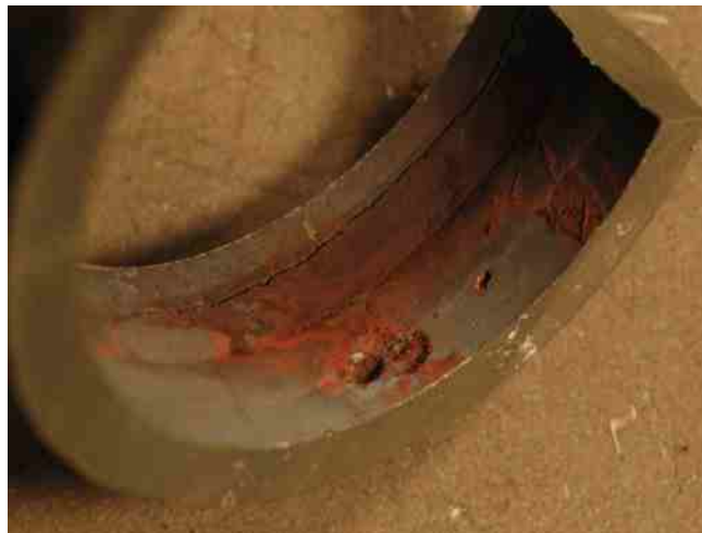
Figure 5-1: Pitting and Stress Corrosion Cracking
