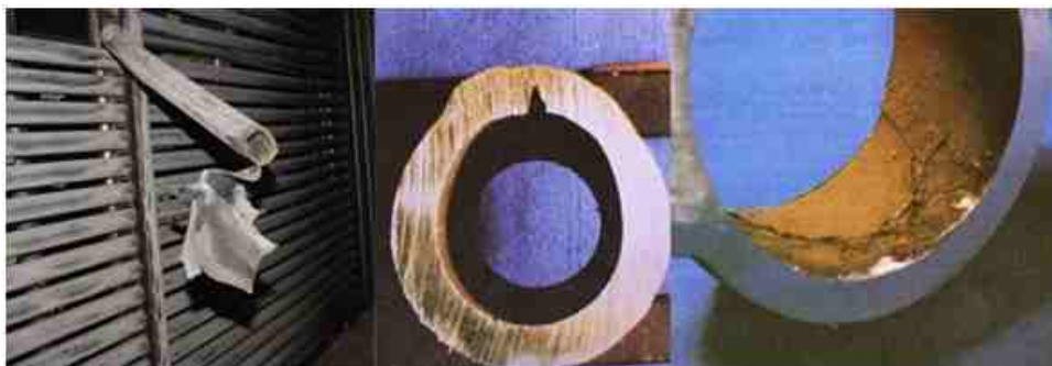
Figure 9-45: Weld and Repair Defects
